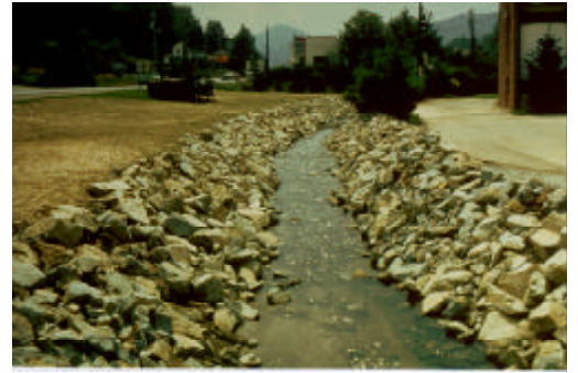
A. Riprap solves the erosion problem at the expense of the stream's natural beauty.
