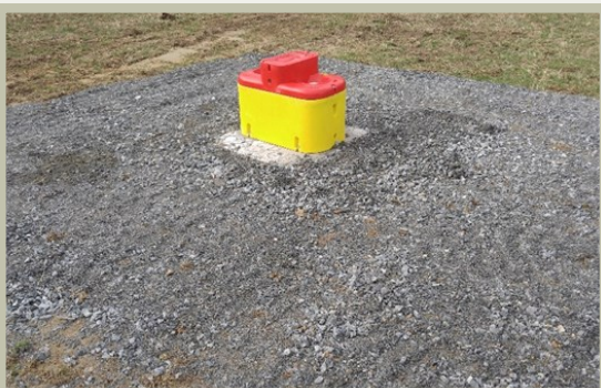
Livestock watering tank with heavy use area protection
