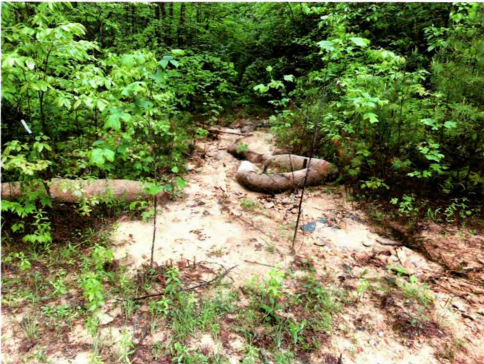
Photo 10 – View of an example of a failed sediment and erosion control which is contributing to sedimentation in Stream H (Perennial).
