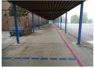
Drop off area with profiled metal awning structure and damaged poles.
