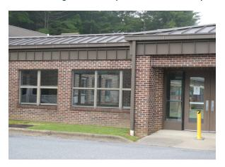
Brick masonry exterior wall and aluminum framed windows
