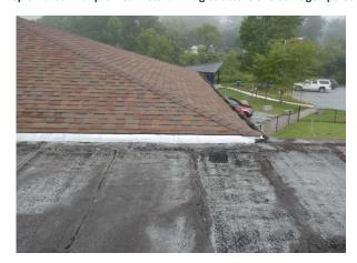
Asphalt shingle and modified bitumen low-slope roof
