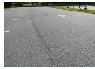
Asphalt with alligator cracking
