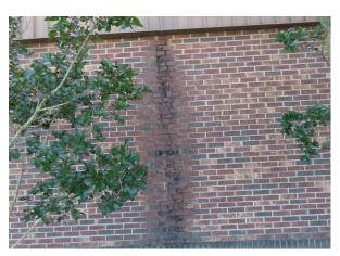
Exterior brick masonry and staining to brickwork
