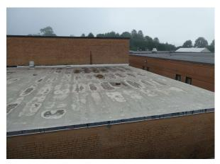
Roof covering at EC Wing in poor condition
