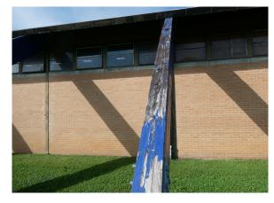
Deteriorated paint finishes at glulam beams at Old Gym
