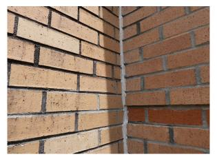
Sealant joints in brickwork in poor condition
