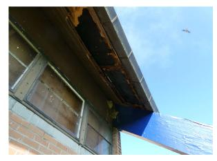
Failed and missing roof deck at Old Gym
