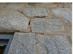
Cracking and deterioration to mortar joints
