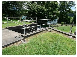
Missing handrails (right and left of steps) at change in level
