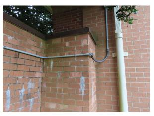
Exterior brick masonry with deteriorated sealants and spalled brick
