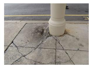
Typical concrete panel sidewalk damage extending around column
