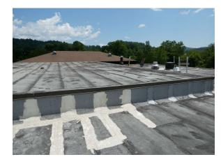
Deteriorated modified bitumen roof and previous repairs
