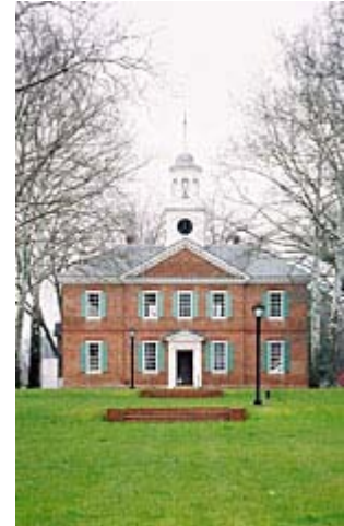
The Chowan County Courthouse, constructed in 1767, outdates the birth of the United States. It is the oldest government building in the state and the most intact colonial courthouse in the country. (Photo courtesy John Ed Whitehurst)
